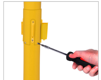
Step 1: Remove post retaining screws
